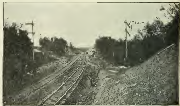
FIG. 11. RIGHT-HAND TRACK, TWO BLOCKS IN ADVANCE CLEAR—PROCEED.
